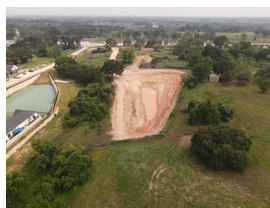
D22A Eastside Tributary Drainage Improvements
